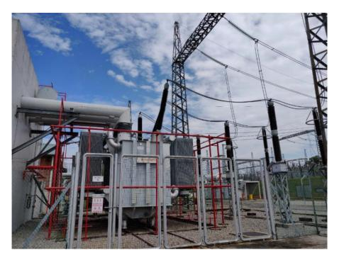
15kV / 6.9kV Step Down Transformer
